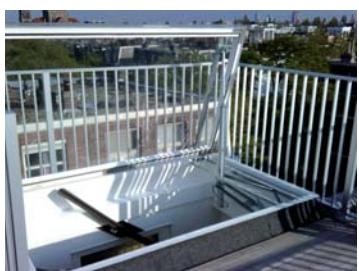
Roof access hatch with electric operation
