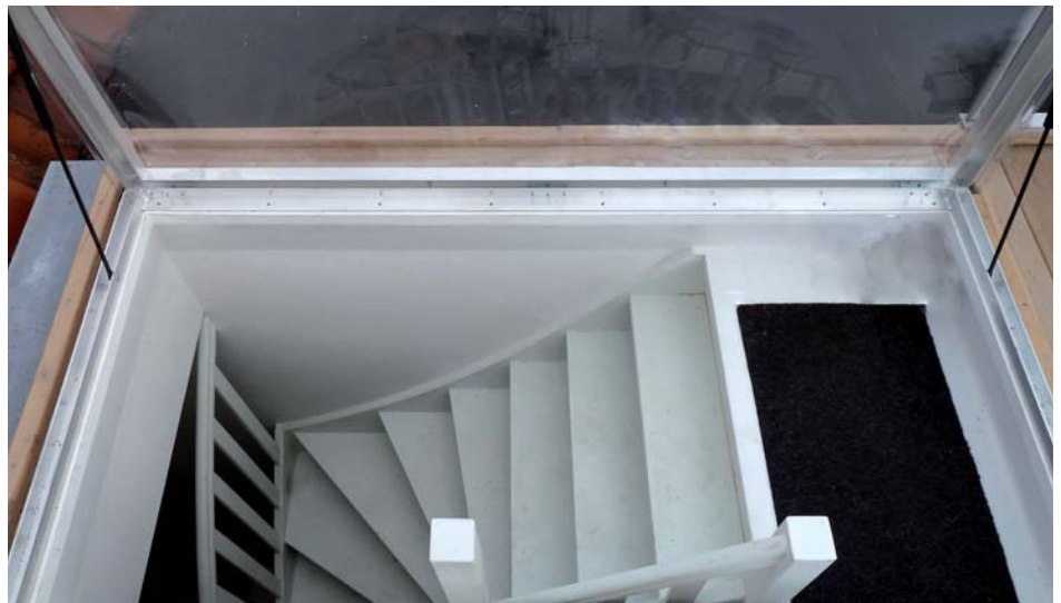
Roof access hatch, aluminium frame with gas springs, crank and handle
