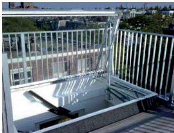
Roof access hatch with electric operation
